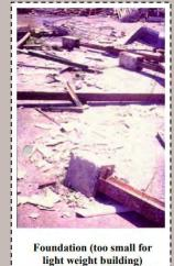
Foundation (too small for light weight building) pulled completely out of ground
